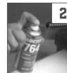
2. Spray Loctite Primer in and around the cable end to thoroughly remove grease and grime.
