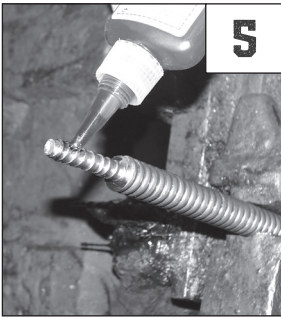
5. Apply Loctite Retaining Compound to other end of splice core.
