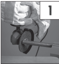
1. Cut the cable end and remove any burrs with a grinding disk or file.
