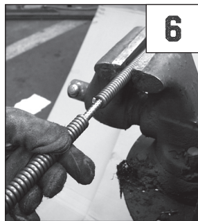
6. Align other piece of cable onto splice core.
